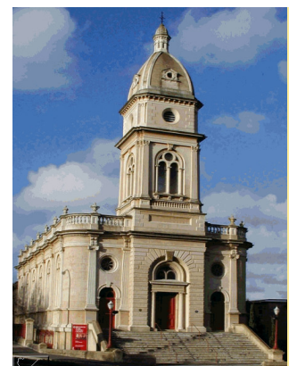
Brougham Place Uniting Church
