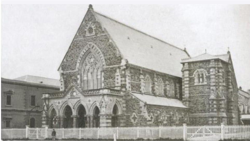
Stow Memorial Church (now Pilgrim Uniting Church) photog. c1900
